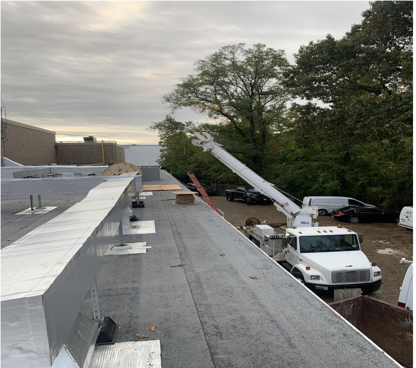
Jr/Sr HS New Addition Electric Service Wiring
